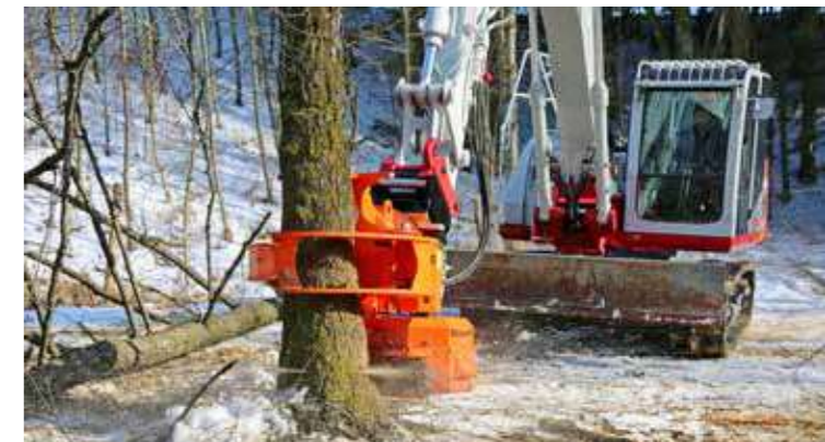
Rapid chopping and piling.
