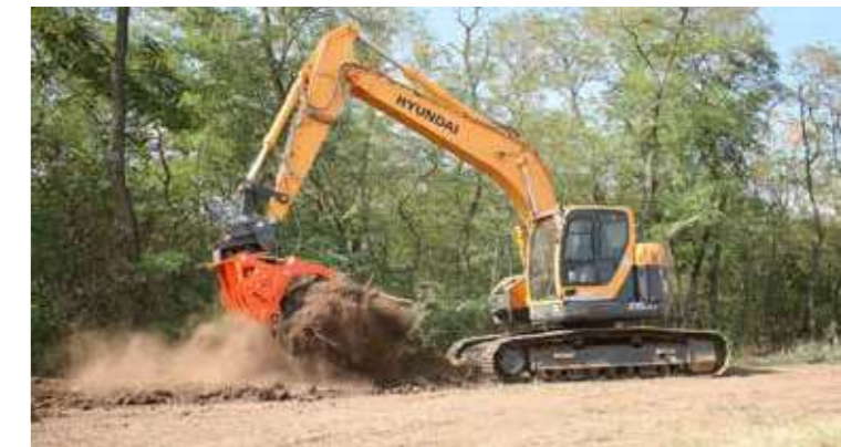
Clearing and caring of large areas.
